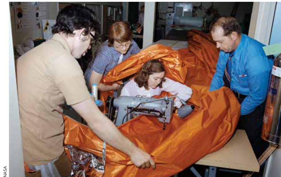
When Skylab's heat shield was damaged during its uncrewed launch on May 14, 1973, NASA scrambled to find a fast solution. Alyene Baker (center) stitched a replacement that a crew carried into space nine days later, just in time to save the space station.
